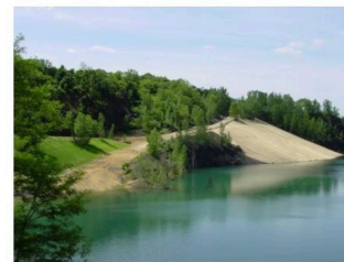
View of the erosion control matting installed on a 2:1 slope after cutting and regrading.
