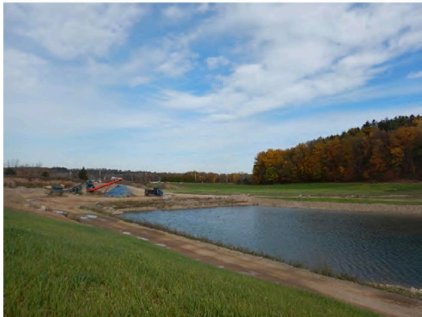
Photo 12 – Rolling Hills Pond Mine – Concurrent reclamation of side slopes around the pond, with active mining occurring in background.
